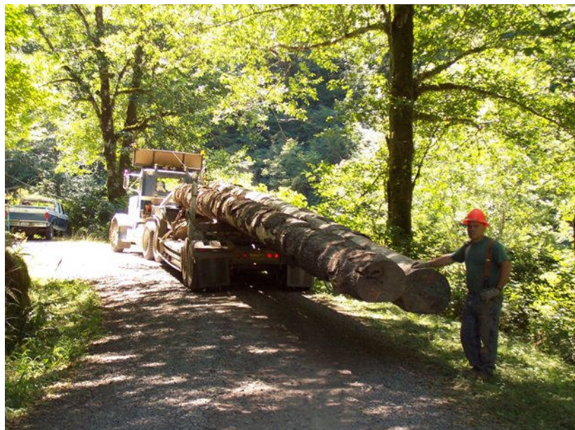
70-foot long logs to be placed into Elk Creek.
