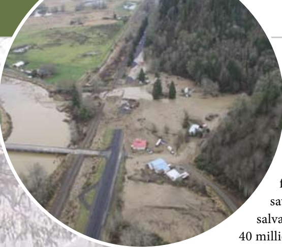
▲ A debris flow at Eilertsen Creek near the community of Woodson brought an estimated 40,000 cubic yards of mud, water and debris down onto the highway and nearby homes and businesses.
