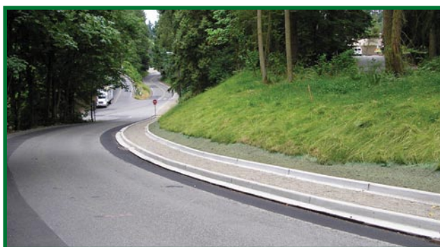
Roads used a 50 percent blend of slag cement in a sidewalk project
