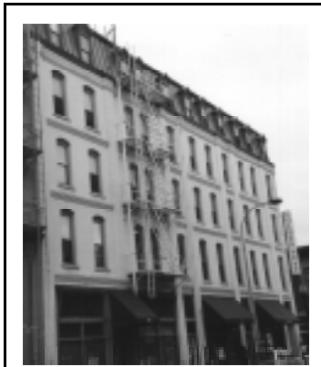
A single room occupancy SC site
