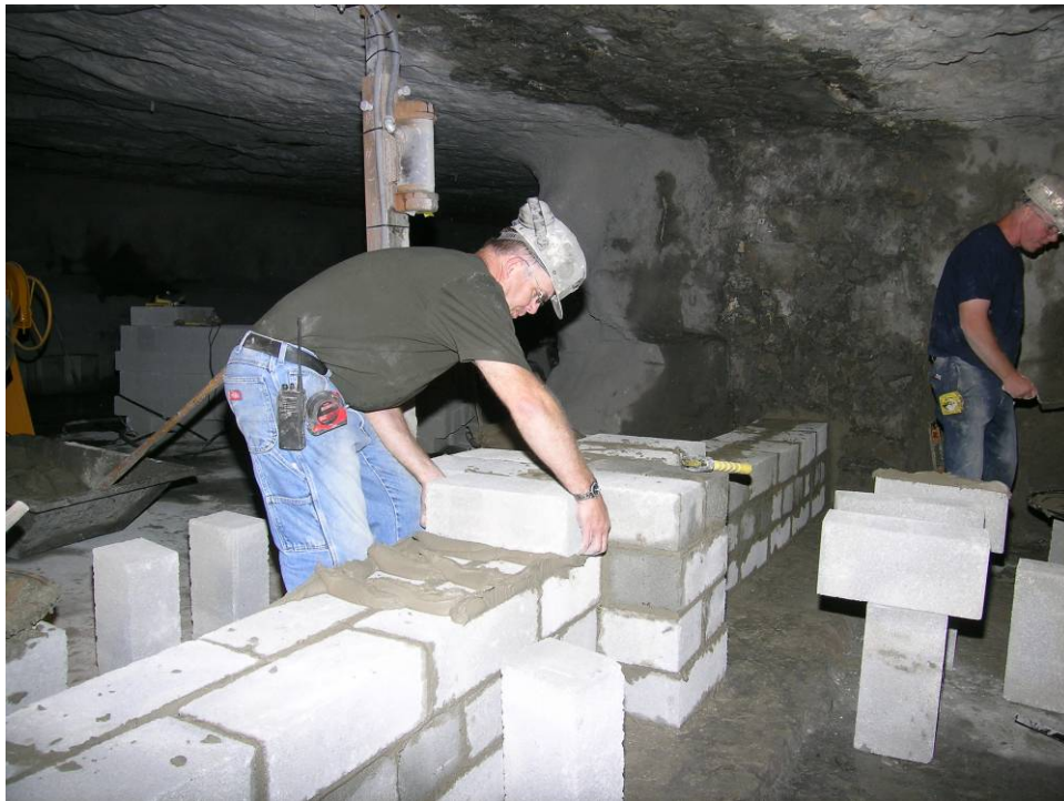
Figure B6-1.-Full wet-bed construction on all horizontal and vertical block joints.
