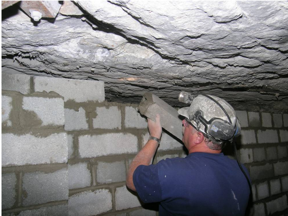
Figure B6-2.-Installing cut block to on top course.
