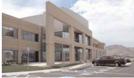
Jefferson County Workforce Center's new building located in Golden, Colorado.
