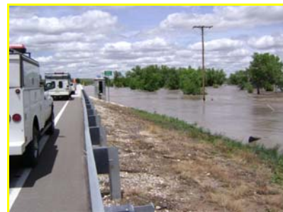
Fig. 4. Flood waters along Wolf Creek at Lipscomb.
