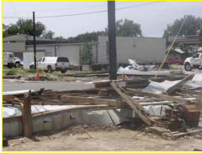
Fig. 5. Remnants of a lumber yard in Miami, Texas.
