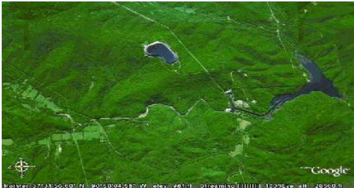
Figure 1-2. Pre-event satellite photograph showing the upper and lower reservoir, the powerhouse and the East Fork Black River along the Johnson Shut-Ins State Park. (Source: Google Earth, 2005)
