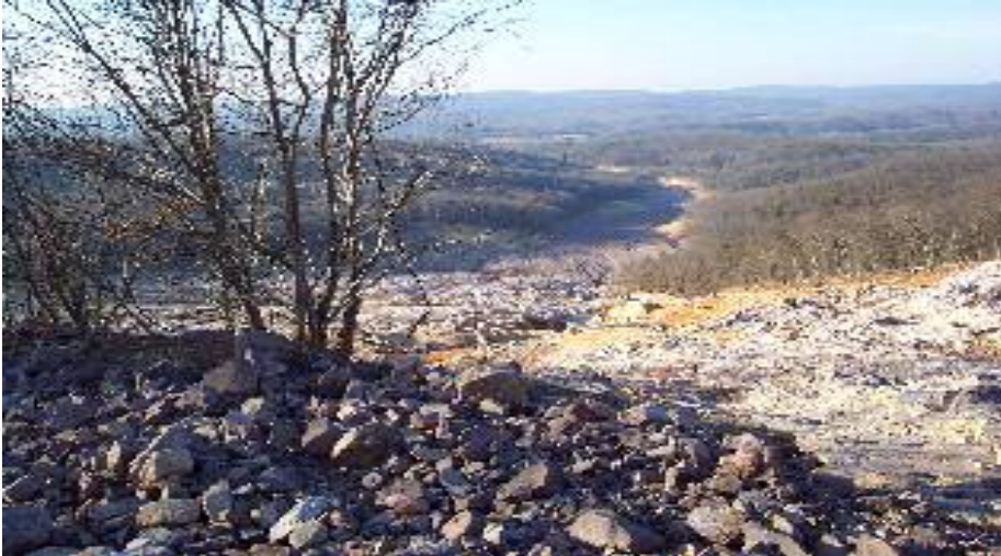
Figure 5-7. Downstream view from breach. (Source: FERC Staff)
