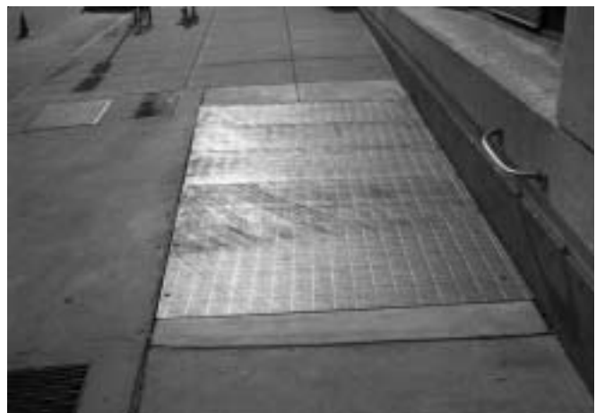
Figure 4. New Grate System
