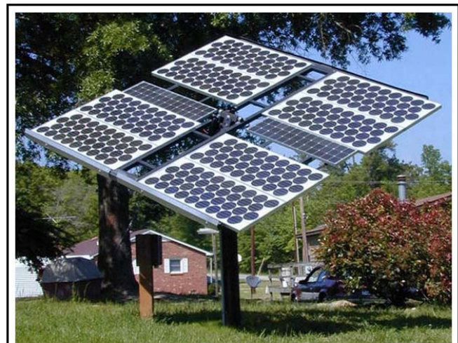
Figure 2-7. Photovoltaic Flat Plate Collector.
