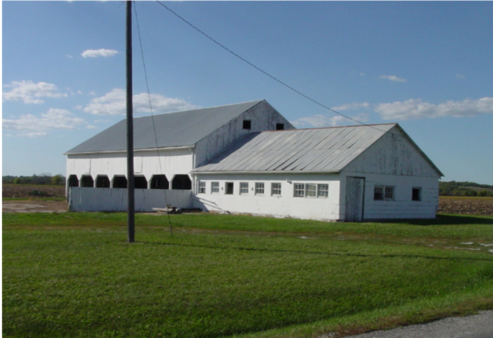
Photograph 3. Outbuildings on North Side of House
