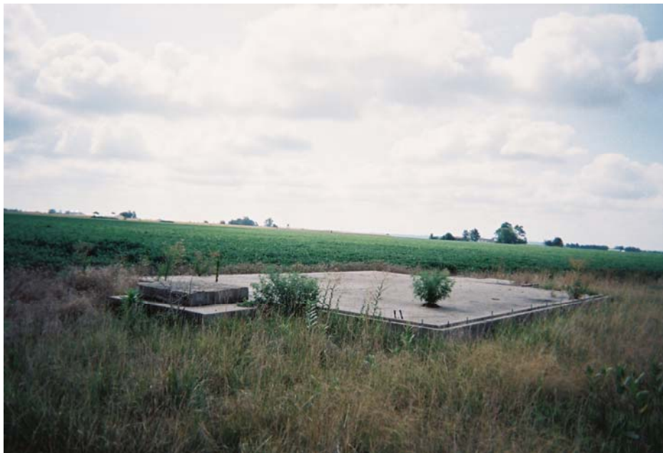
Photograph 7. Farmstead 3 – concrete house slab
