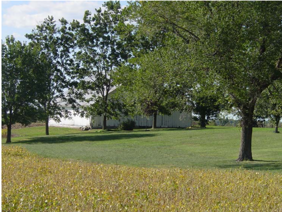
Photograph 5. Barn West of House
