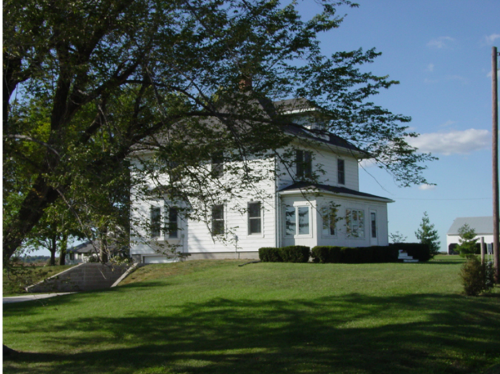
Photograph 1. Farmstead House – view to northwest
