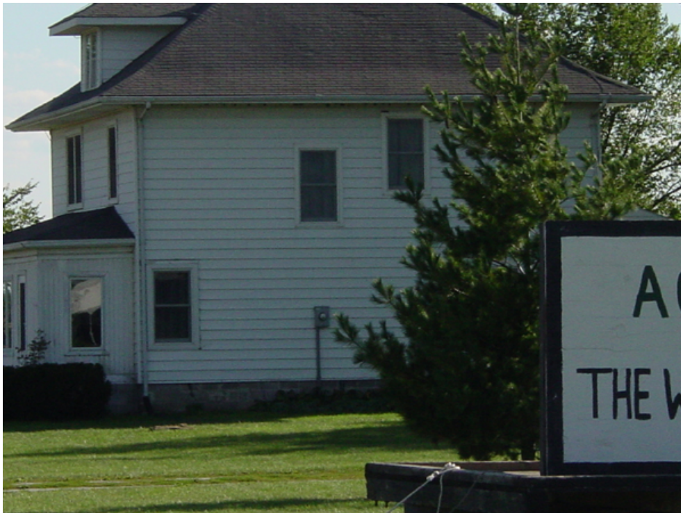
Photograph 2. Farmstead House – close-up showing concrete block foundation & newer siding
