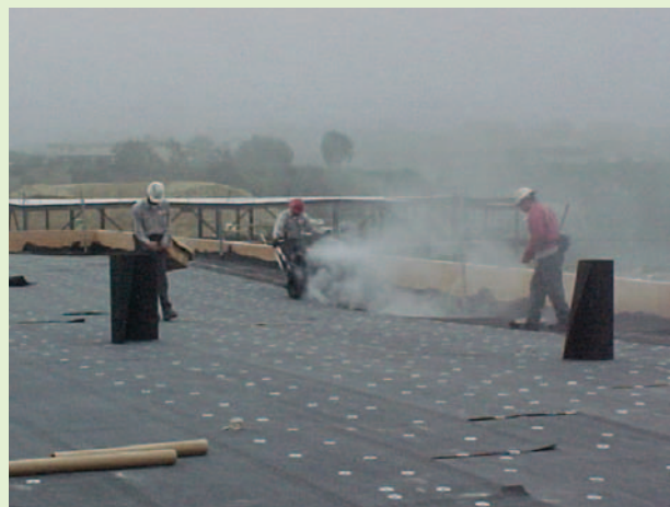
Figure 1. Applying hot asphalt to fiberglass felt.
