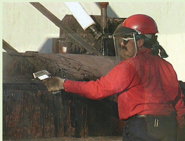
Figure 2. Kettle Operator. Courtesy of Thomas R. Shanahan, National Roofing Contractors Association.
