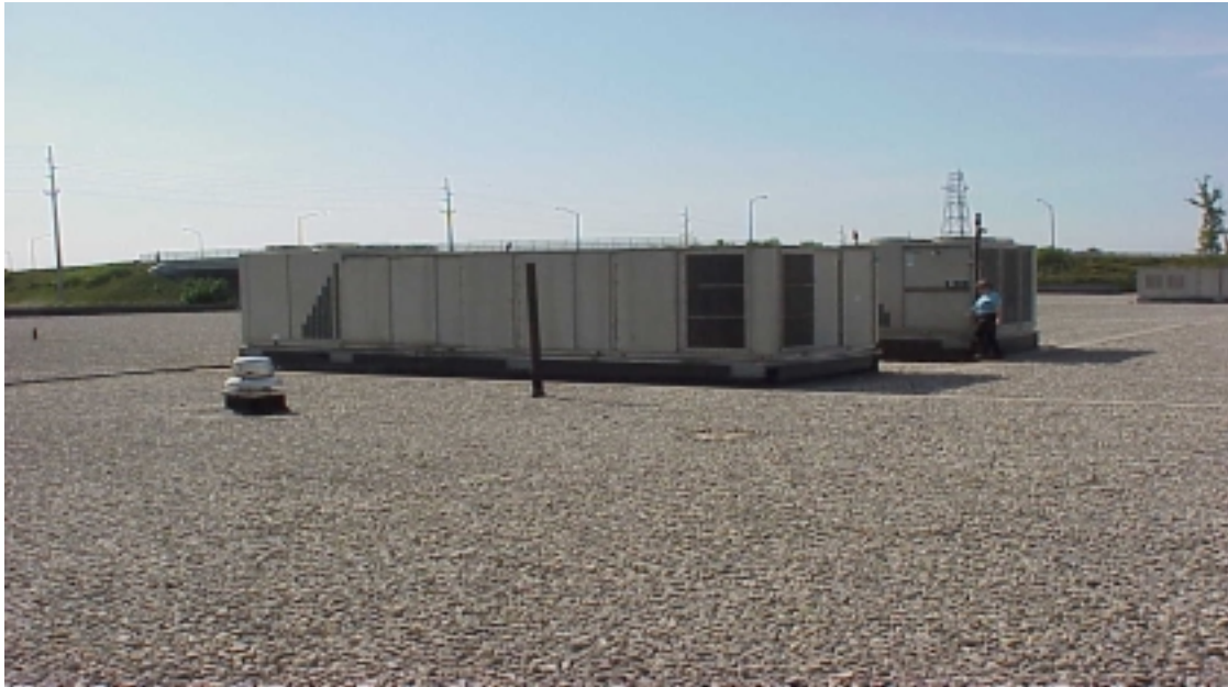
Figure 1. Bathroom exhaust near outside air intake.
