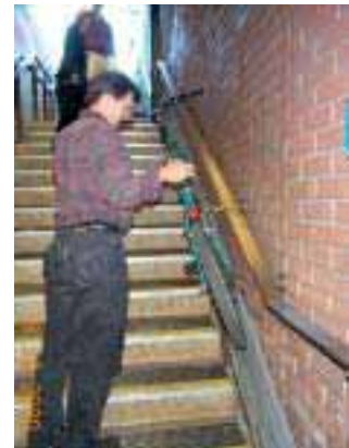
Stairchannel at Downtown Berkeley Station
