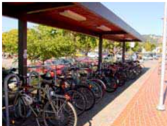
Parking Canopy at North Berkeley Station
