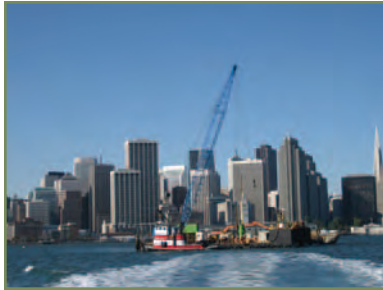
Earthquake Safety Retrofit Construction Barge floats over Transbay Tube
