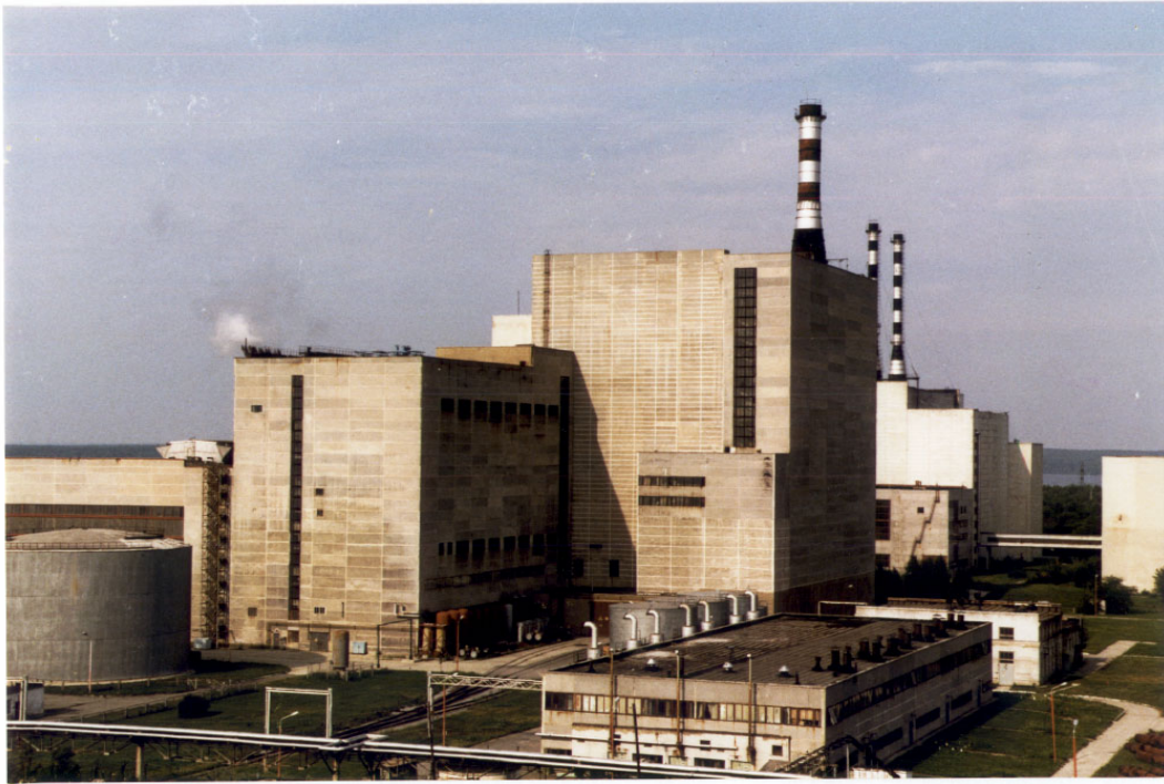
FIG. 3b. The BN-600 power plant building.
