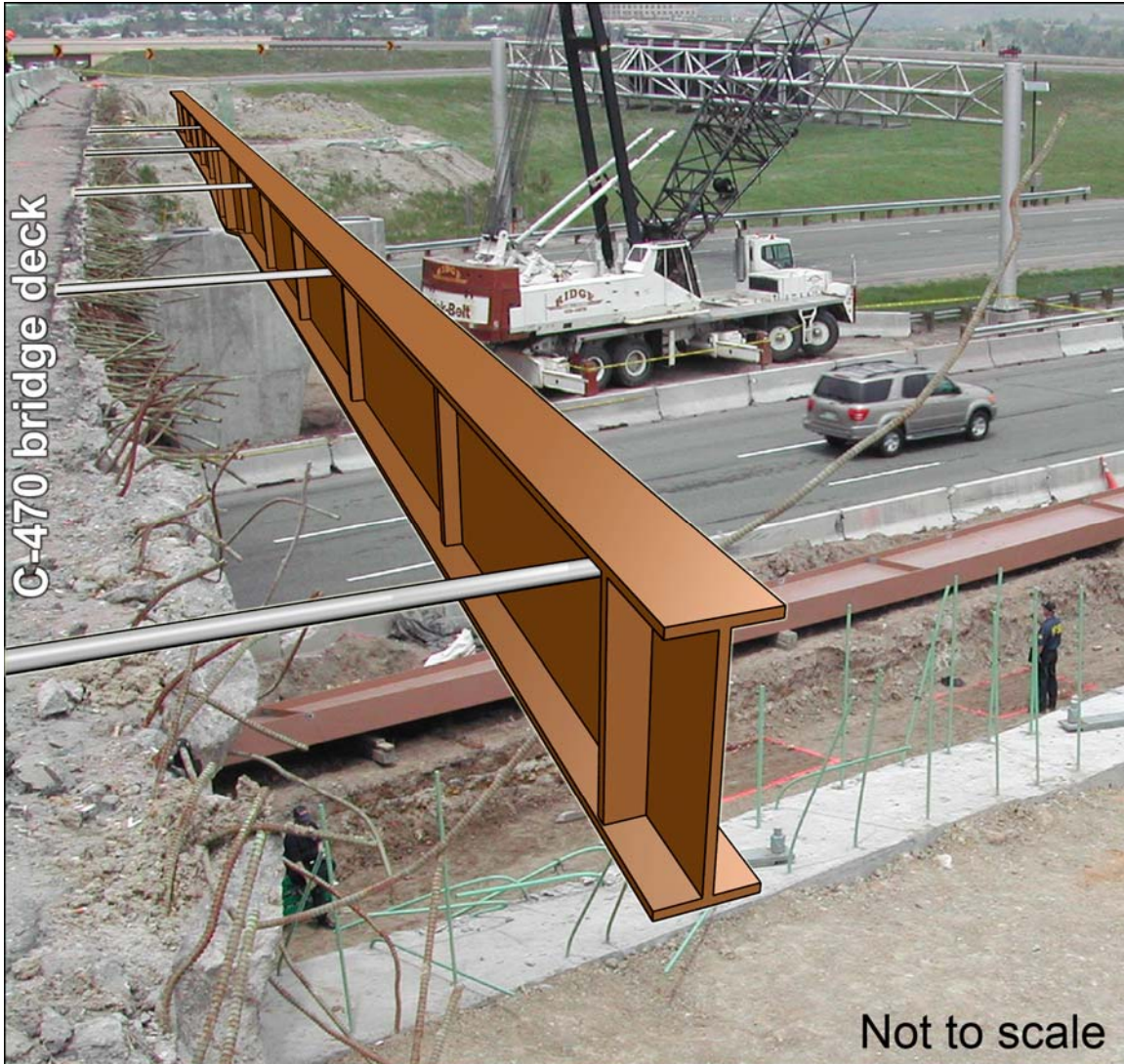
Figure 4. Diagram overlaid on photograph to show the accident girder and five braces in relation to the existing C-470 bridge deck. Note that this graphic is representative only of the approximate relative positions of the girder, bracing, and deck.
