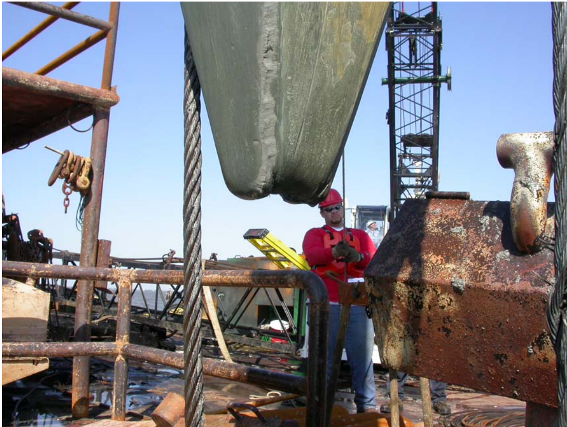
Figure 12. Aft spud of the Athena 106 when raised after it had released from its fully raised position and hit a submerged, buried high-pressure natural gas pipeline.
