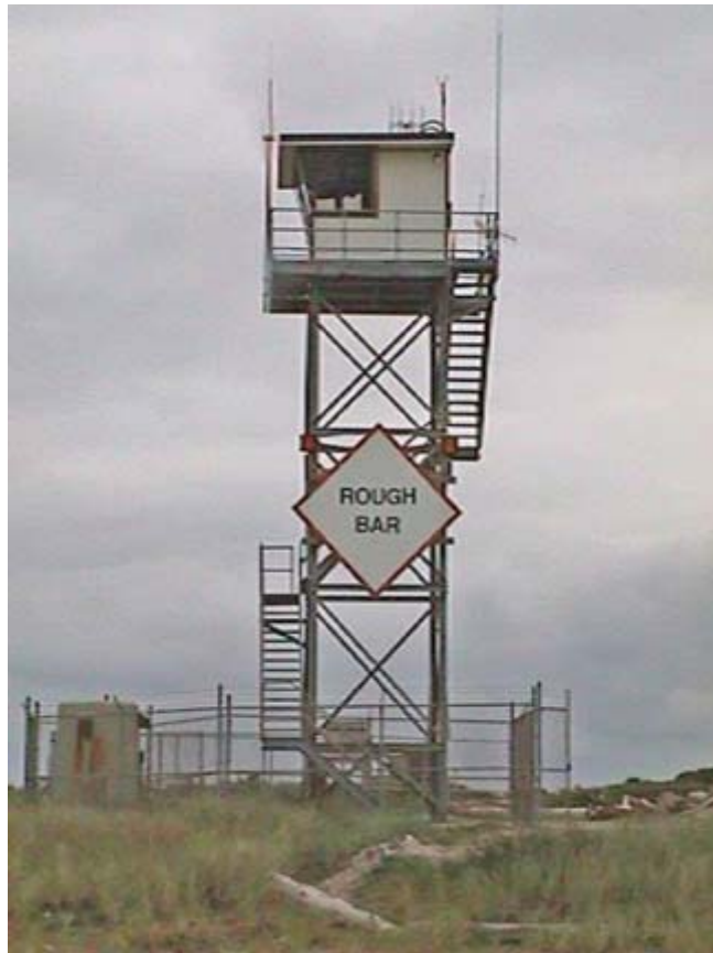
Figure 6. Rough bar advisory sign on Coast Guard observation tower at Tillamook Bay.
