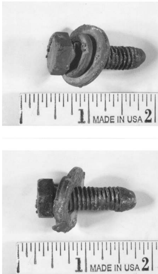
Figure 12. Bolt found on front (aft side) framework of switchboard.
