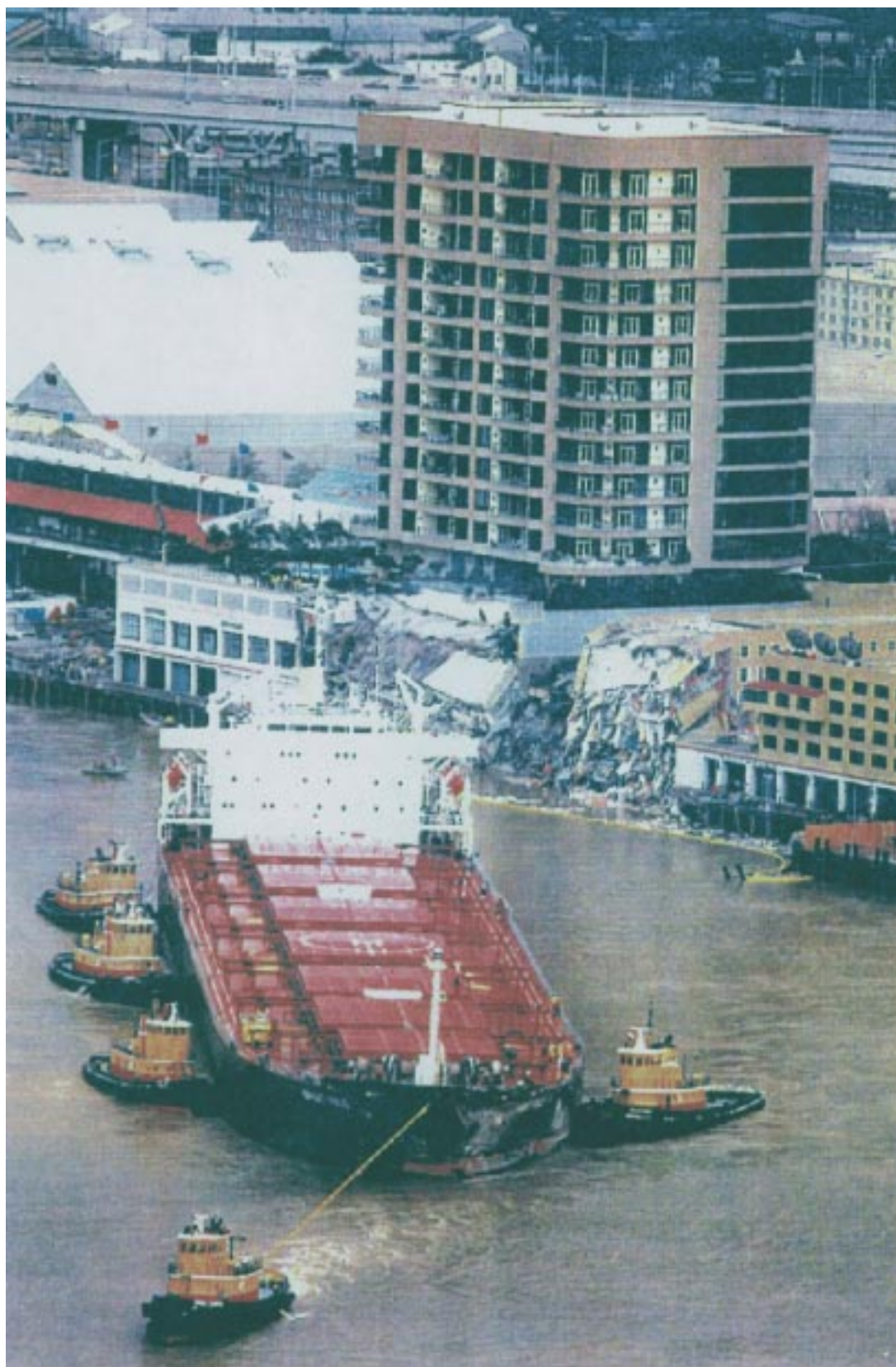
Figure 7 -- Damaged Bright Field being towed away from Poydras Street wharf en route to repair facility, January 6, 1997
