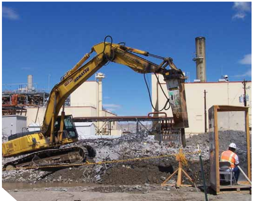
Workers demolish facilities in the N Reactor area.
