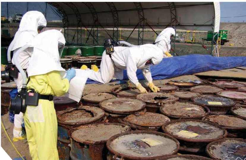
Workers inspect severely corroded waste drums retrieved from burial grounds.
