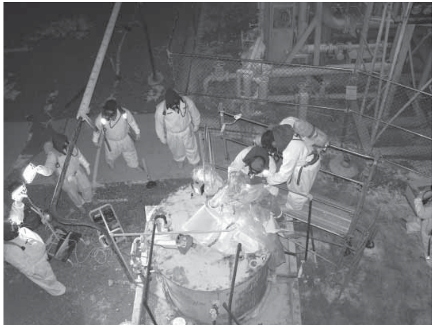
Workers perform a tank inspection.
