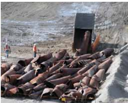
Disposing of N Reactor steam transfer lines in the Environmental Restoration Disposal Facility (ERDF).
