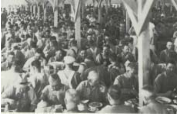
Construction workers at one of eight mess halls
