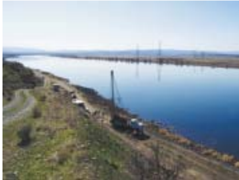
Groundwater remediation workers drill monitoring wells along the Columbia River
