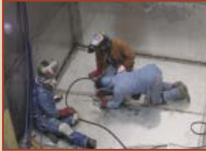
WTP Low Activity Waste Facility
