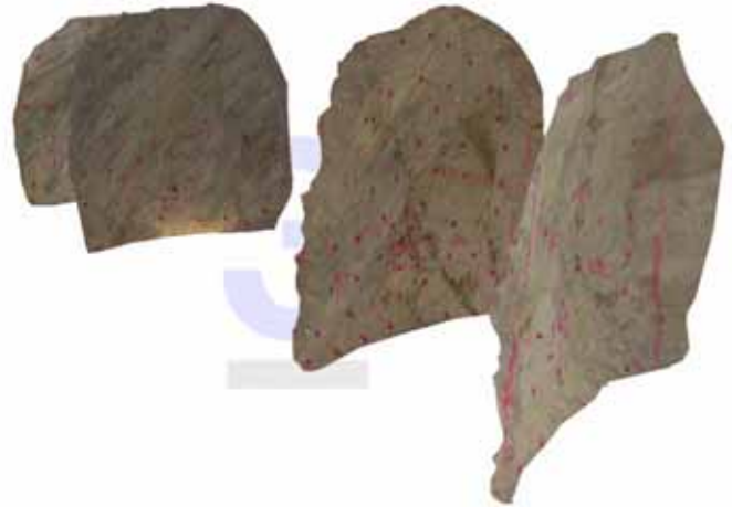
Figure 26: Subsequent 3D images of drift tunnel excavation in an underground mine. The marked points represent the borehole positions that were measured together with the geometry of the tunnel face and the geological conditions.
