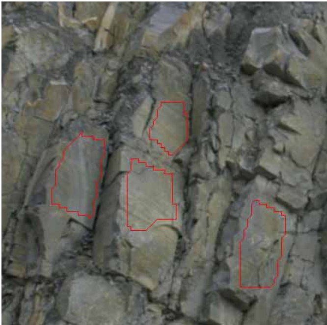
Figure 9: 2D image of the measured discontinuity planes
