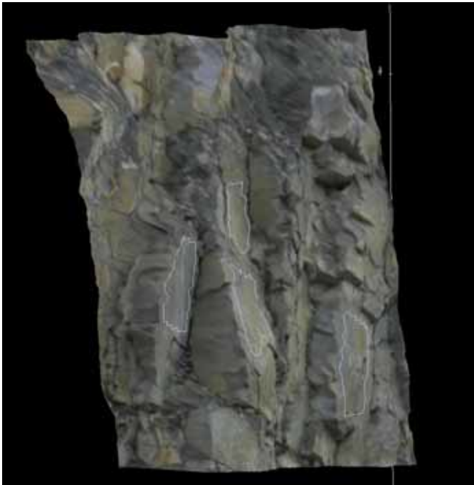
Figure 10: 3D image of the measured discontinuity planes
