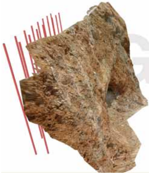
Figure 25: 3D image of a bench face in a quarry and planned borehole positions. The system provides the blasting engineer with the required geometric information on the rock wall, as well as the distance between boreholes and surface (burden).
