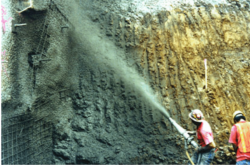
Figure 14. Shotcrete Technologies nozzle being used for concrete gunning.
