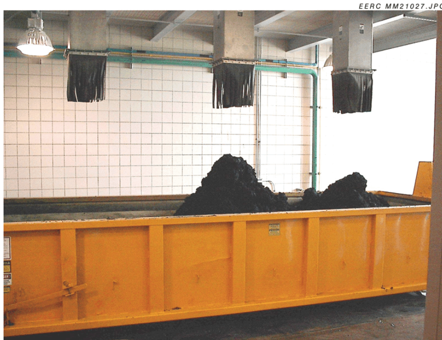
Figure 1. Fargo municipal sewage sludge discharging from belt-filter press.
