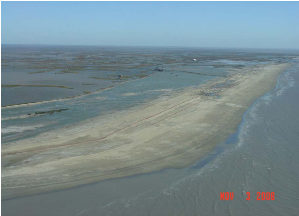
Figure 5-3. Barrier Island Project Nearing Completion in Fall 2006
