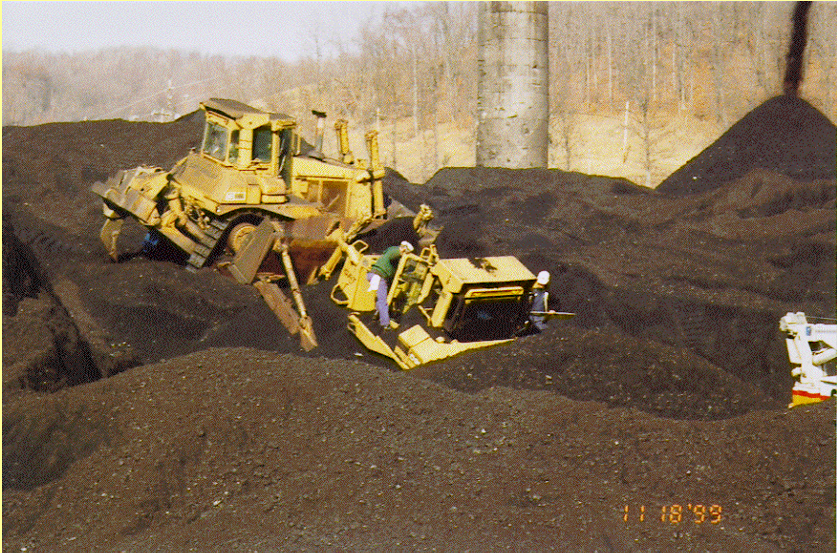
Checking windows after burial.
