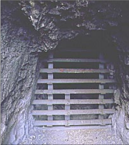
▲ The Socorro West Mine Safeguard project outside Socorro, New Mexico reclaimed abandoned mine shafts, adits, and stope openings. Because the mine workings were home to a large population of bats, gates were constructed that allow ventilation and bat entry; but, keep people safely out.
