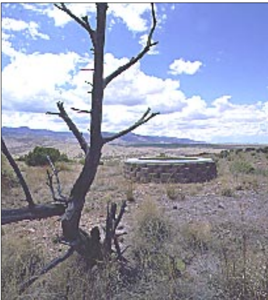
▼ The dangerous open vertical shafts have been covered with bat gates and people who visit the site no longer have to fear they will fall into an open mine shaft. With public ownership and good rock-climbing opportunities in the area, the land around the mine site is used for both cattle grazing and recreation.
