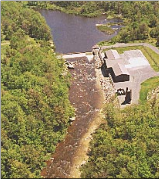
▲ The Blackwater River Limestone Drum Station has eliminated acid mine drainage in this West Virginia river. Much of the coal mining along this stream occurred during the 1960's, before passage of the Surface Mining Law and when there was very little mine reclamation completed. The station provides treatment with a rotary drum system that uses six water-powered cylinders to grind limestone aggregate into a slurry. As the river's flow changes the drums automatically adjust their slurry output.
