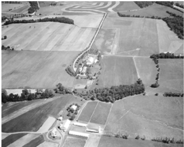
At Eisenhower National Historic Site, the significant characteristics and features of the cultural landscape have been inventoried and included in the NPS Cultural Landscapes Inventory.
