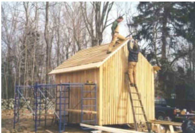
Corn crib restoration at Weir Farm National Historic Site.
