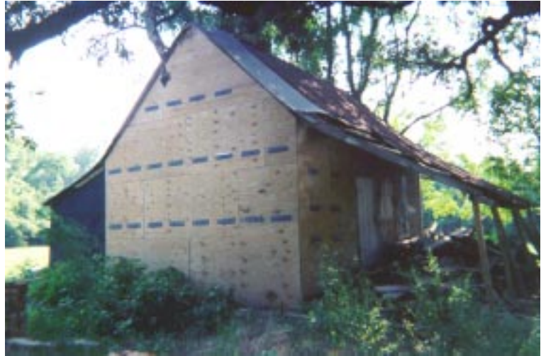
Slave home on Oakland Plantation at Cane River Creole National Historic Site stabilized until restoration is funded.
