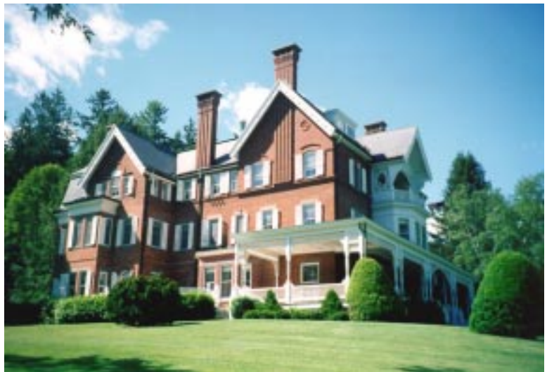
Exterior view of the residential mansion at Marsh-Billings-Rockefeller National Historic Park.
