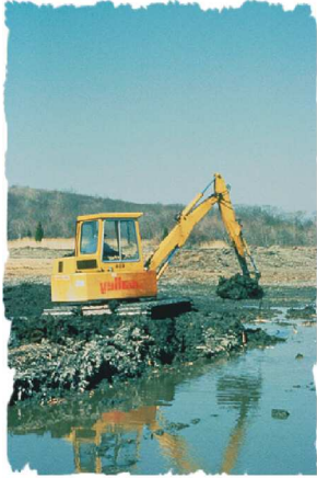
Coastal marsh restoration
