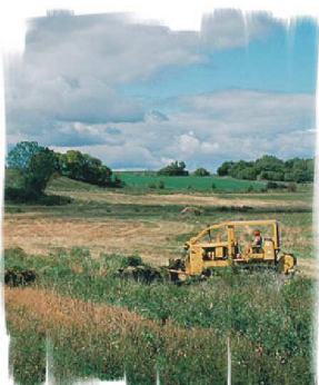
Lower levee to restore wetlands
