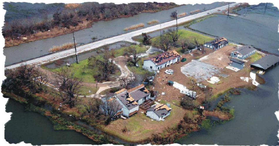
Sabine NWR from the air showing roof damage and huge pile of debris
