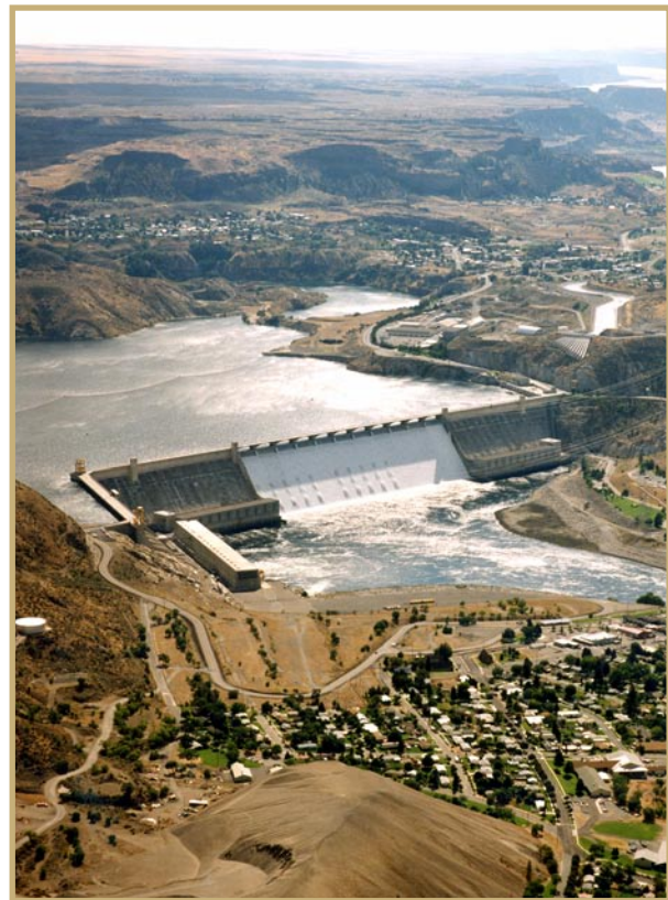
Integrated security upgrades have been completed at Grand Coulee Dam, located on the Columbia River in Washington.
