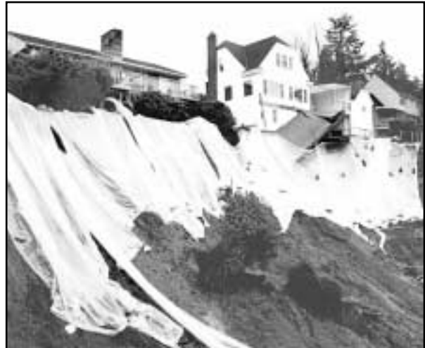
Landslide at Magnolia Bridge, Seattle, Wash. The porch at the back of the light-colored house was undermined and collapsed. The head of the landslide was covered with plastic sheets to prevent additional rain water from entering the slide.
