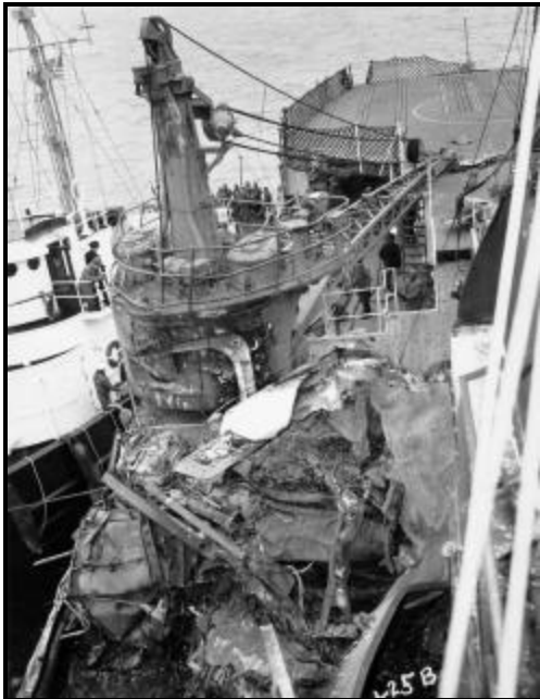
View of damage to the starboard side of the CGC EASTWIND
