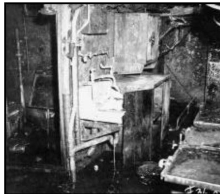
Fire damage to the Chief's Quarters
