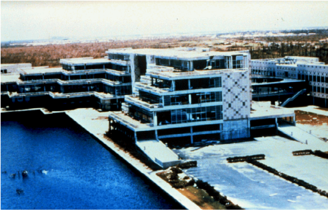
An aerial view of the World Headquarters for Burger King, site of a 16.9-foot storm surge. Note the windows blown out by Andrew's intense winds.
