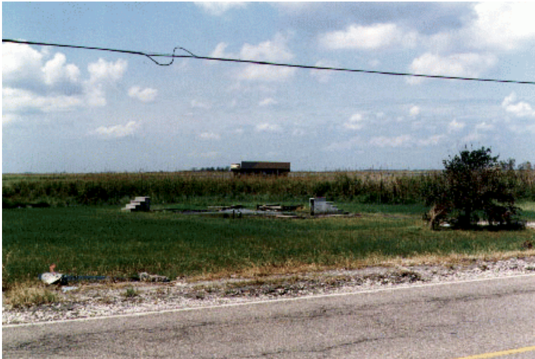
North of Cocodrie, Louisiana, home in the background was removed from its foundation by a combination of storm surge and wind.
