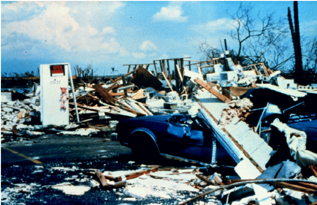
Naranja Lakes homes destroyed by Andrew's devastating winds.
