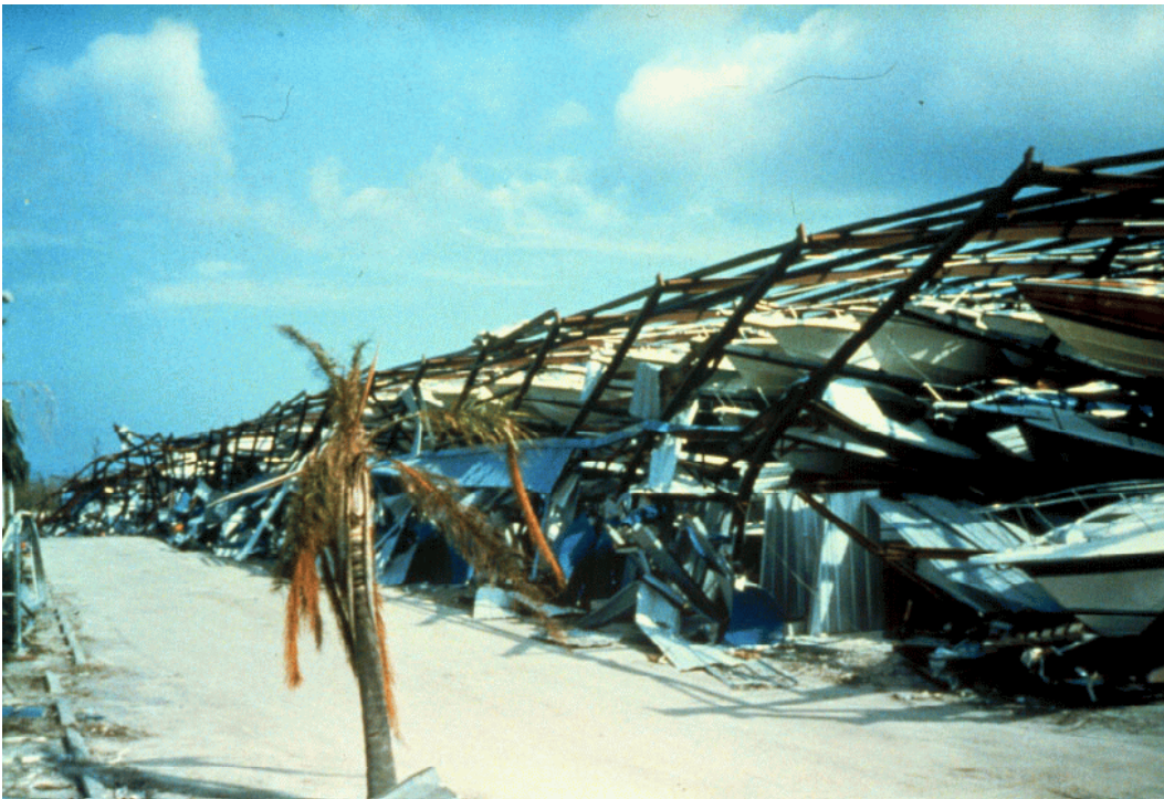
This stack storage facility at Black Point Marina, Dade County, collapsed under Andrew's intense winds. One-third of the 45,000 registered boats in Dade County were damaged.
