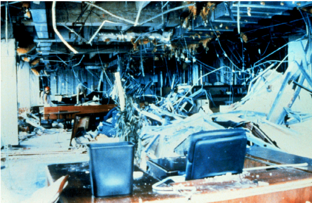
This photo depicts wind damage to the top floor of the Burger King World Headquarters building.
