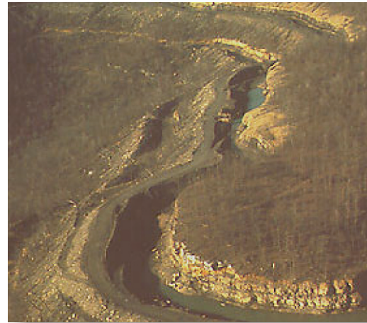
In eastern Tennessee, this photo from the early 1970s shows an unreclaimed contour mine. Without any reclamation, the dangerous unstable highwall is exposed and left to erode and pollute nearby streams.
