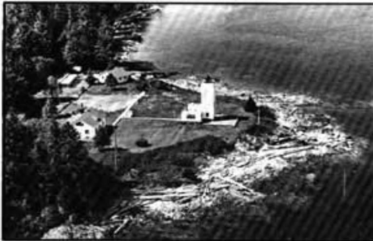
The newer structure at Mary Island in 1965.
