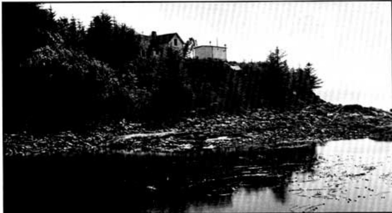
Fairway Island Light Station, 1944.
