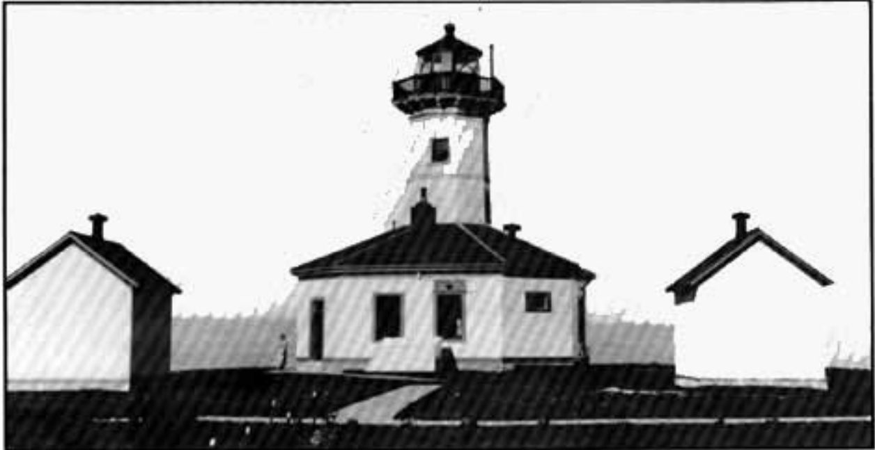
The original lighthouse structure at Mary Island.
