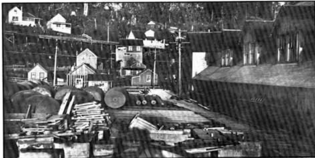
Buoys line the dock at the leased Lighthouse Service depot building in Ketchikan, December 1916.
