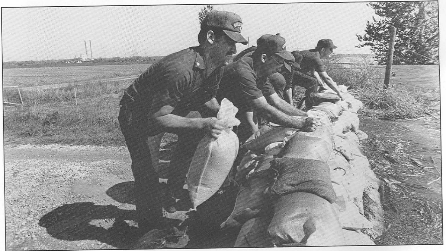
Coast Guardsmen place sandbags along a rising river. Flood duty periodically occurs along the Western rivers.
