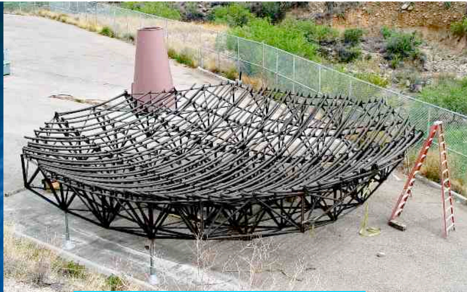
Optical Support Structure Amber Steel, Chandler, AZ
