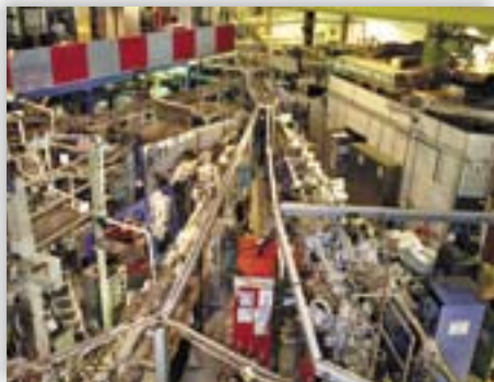
This view of the NSLS experimental floor shows four aluminum-foil-wrapped beam lines. Why foil? For light to travel down the beam lines properly, they are heated to "bake" away molecules attached to their inner walls. Just as with baked potatoes, the foil helps keep the beam pipes hot.
