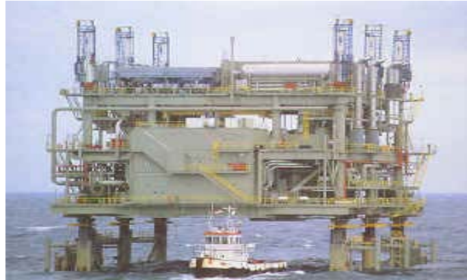
Fig 4. Thorough knowledge of the historical wind and wave conditions at any specific location is crucial to the design of drilling platforms.
