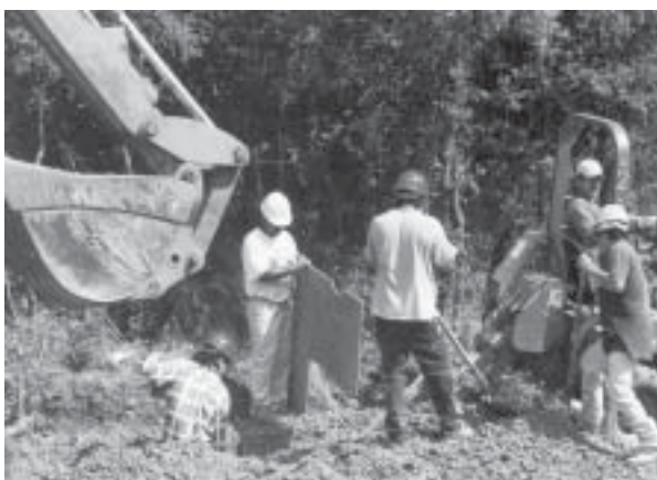
Kennedy Ridge volunteers work on installing their new water and sewer systems.
