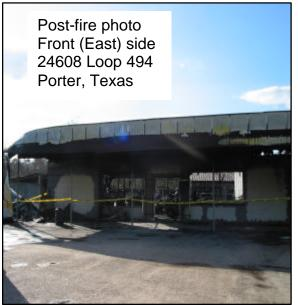
remainder of the building is corrugated metal installed over wood joists supported on metal columns. There is a rear overhanging roof protecting an open storage area enclosed with chain link fencing. There are several additions to the original building.
