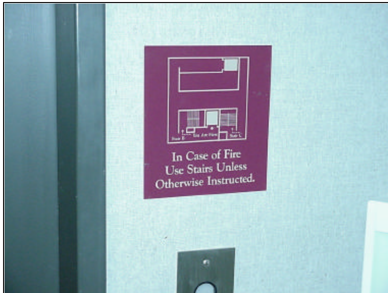
Figure 15-Floor plan sign located in all south service elevator lobbies.
