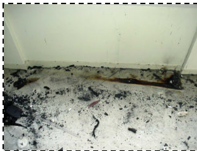
Figure 12-close-up of scorched carpet in dashed area from Figure 11
