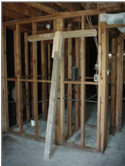
Figure Six. "T"-shaped floor jack found in area adjacent to fire.
