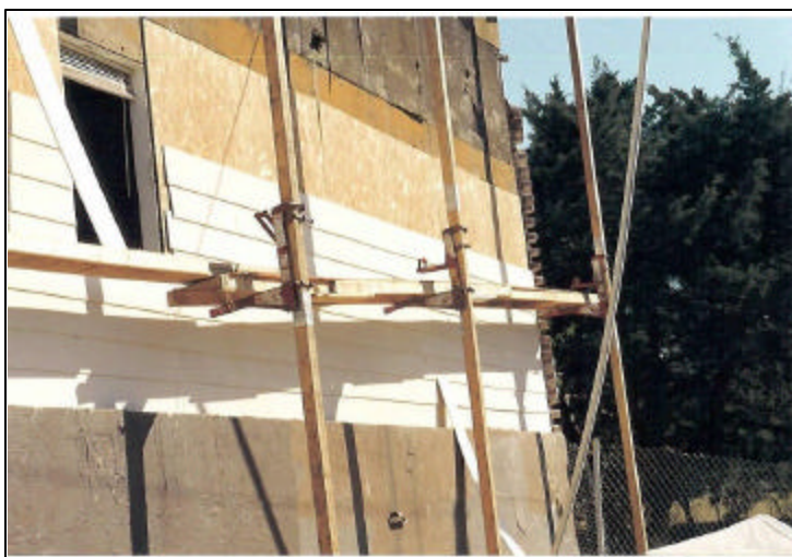
Figure Eight. Southeast end of Section 3 showing brick removal. Photo by BATF.
