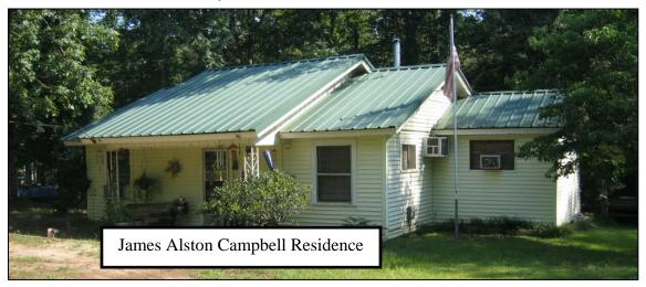
The residential dwelling is a wood frame residence having a pier and beam foundation, an exterior vinyl siding, and a metal roof. The roof system consists of a gable design incorporating gable vents. According to Fire Chief Marc Cummings, the residence is a two bedroom dwelling.
