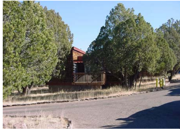
Figure 5 - Vegetation Against Structure
