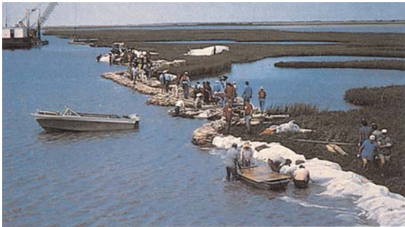
Erosion control efforts along the Intracoastal Waterway at Aransas National Wildlife Refuge © TPWD
