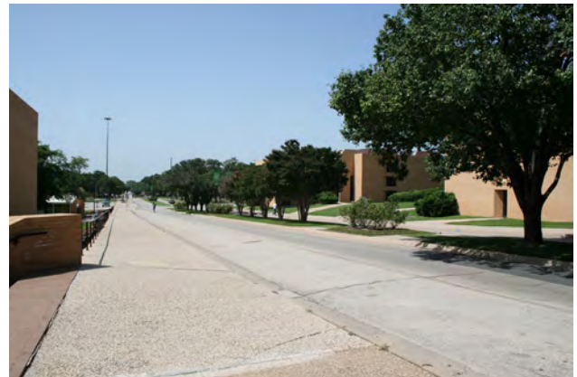
Avenue C - Existing Conditions
