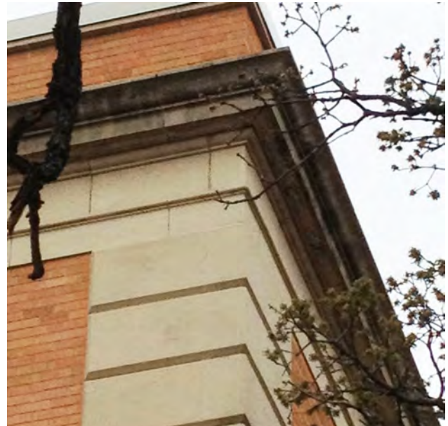
An older building with a flat roof and stone cornice extends the brick parapet and cap for a vertical expression which balances top and base.
