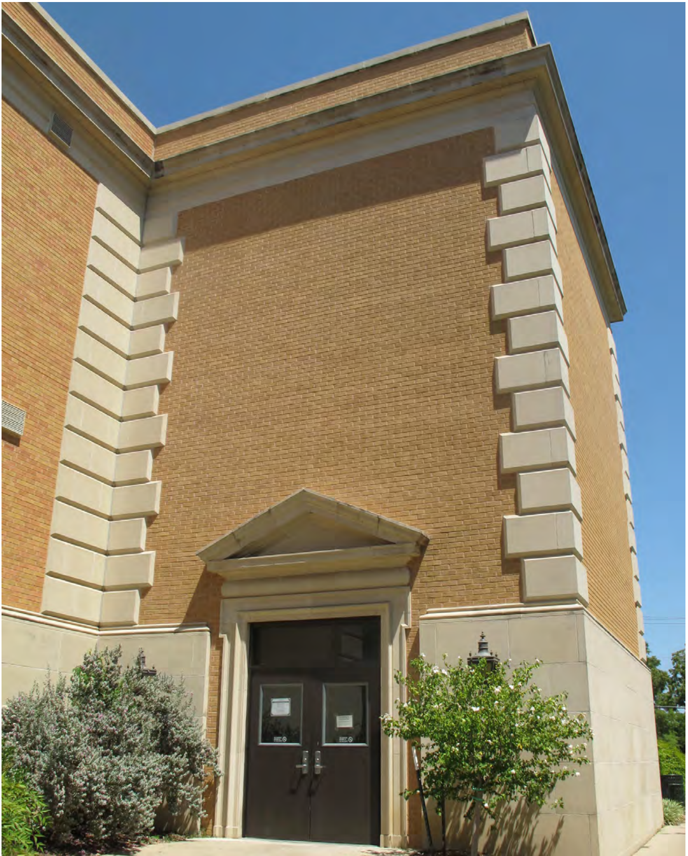
Above is an example of an appropriate expression of the building base, with rusticated quoins terminating fields of brick and defining the building corners; the cornice and extended parapet are seen on many campus buildings. The doorway is given depth and expression with stone trim and pediment.
