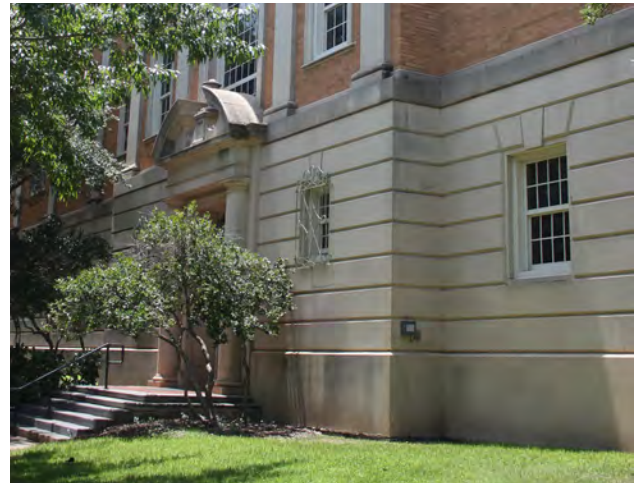
Above are examples of rustication with a horizontal expression, in stone, brick and concrete. Below are examples of quoins and corner bands.
