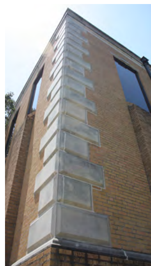
Above are examples of rustication with a horizontal expression, in stone, brick and concrete. Below are examples of quoins and corner bands.
