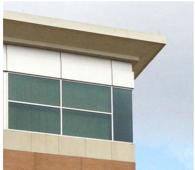
Above is a contemporary cornice, appropriately using a change of materials and depth; on the south side, the extended cornice may shade the windows below.
